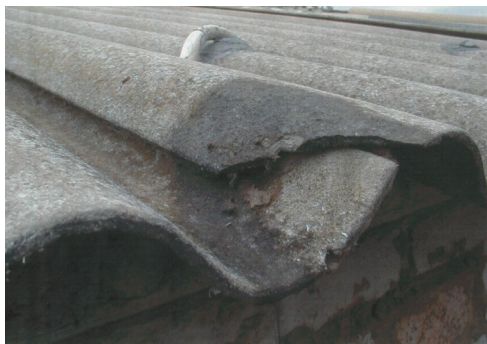
Figure 3. Detail of asbestos roof sheet in Soweto, showing damage and exposed asbestos fibres. (Courtesy of Professor JI Phillips).
